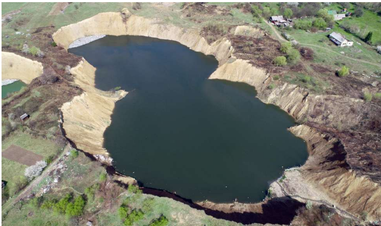
Fig. 2. Flooded mine No. 8
