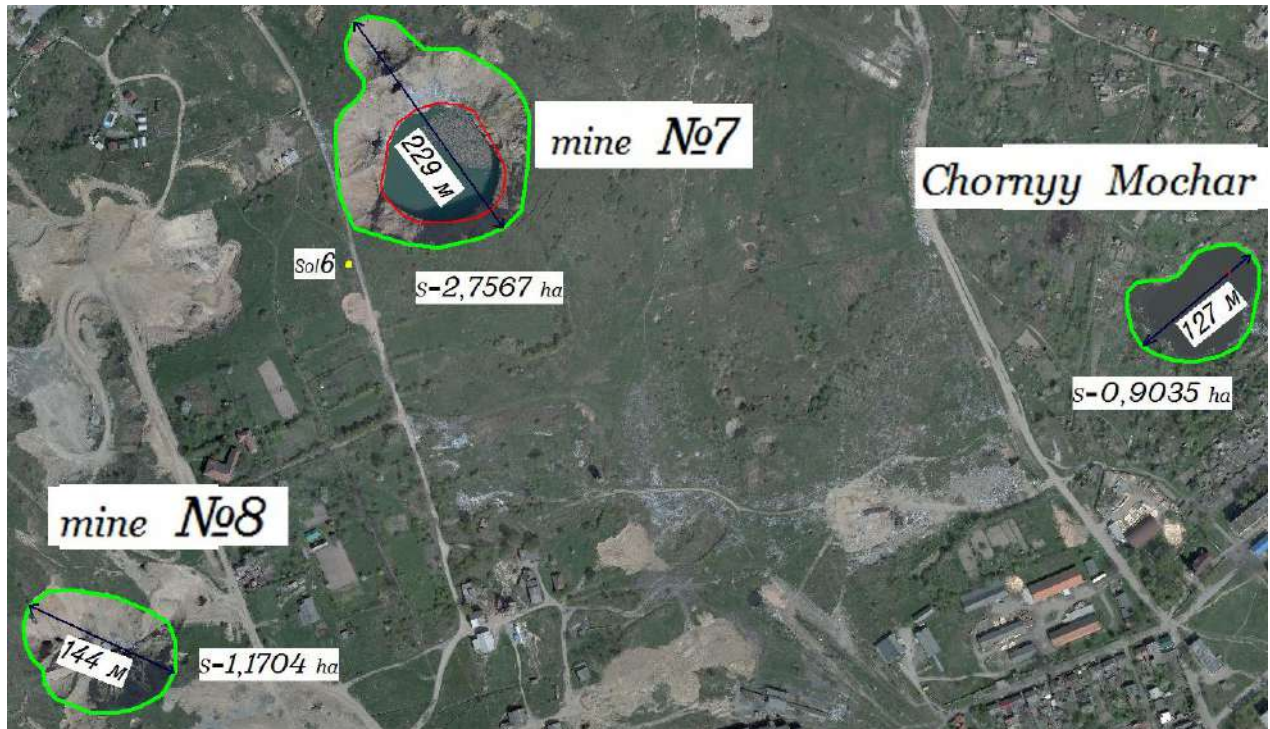
Fig. 5. Monitoring of deformations (aerial photography materials as of 2010) [World Bank Project]
