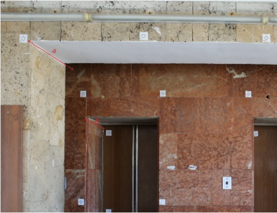
Fig. 3. The depth of the survey object relative to the plane of focus ( a=105 cm; b=50 cm)
