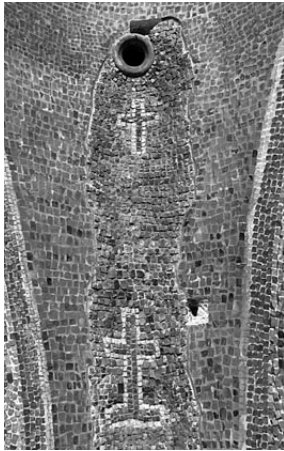
Іл. 9. The resonator hole and images of two crosses in the north-western pendentive
