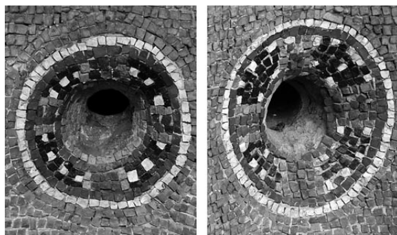
Лл. 8. The resonator holes: in the north-eastern pendentive (on the left); in the south-eastern pendentive (on the right).
