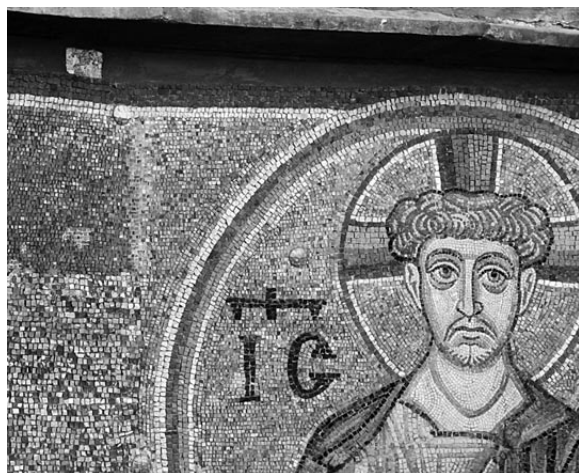
Іл. 20. The under-dome ring, the medallion over the eastern arch with image of Christ the Priest. A light rectangle below the cornice is probe with the remnants of the fresco plaster.
