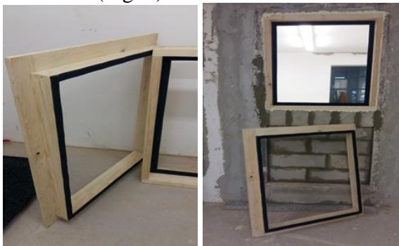
Fig. 1. Installing sound insulation panels during the experiment
