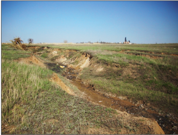
Fig. 1. The earth surface deformations in the territory of Kostenko mine
