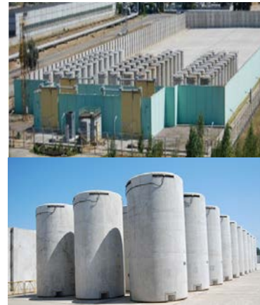
Fig. 6. The dry spent nuclear fuel storage site
