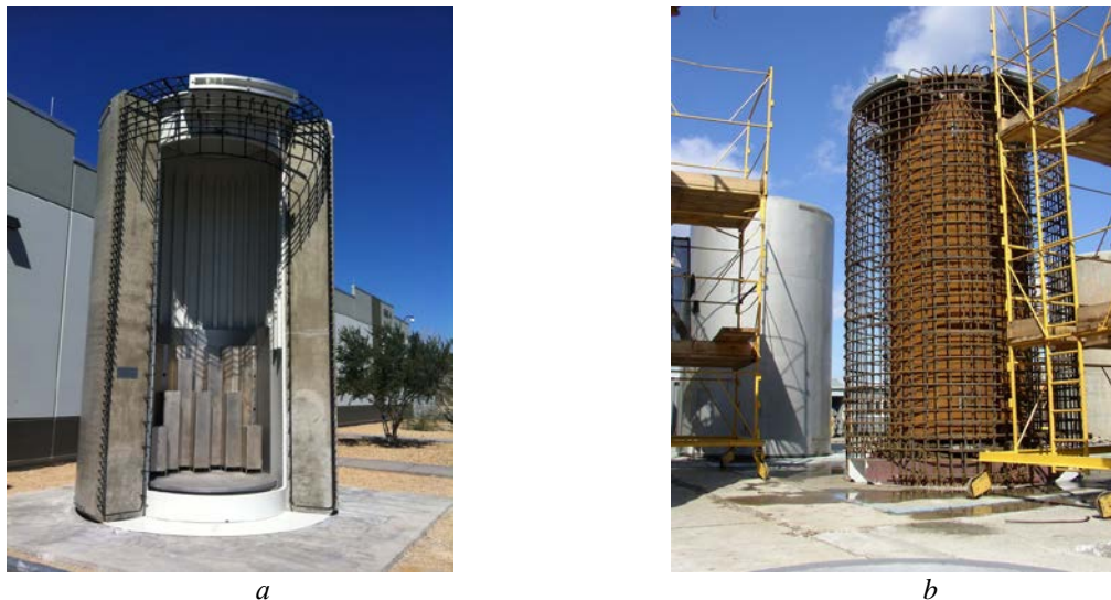
Fig. 4. Design of a container for dry storage of spent nuclear fuel: a multi-seal sealed basket (a), reinforced concrete cask (b)
