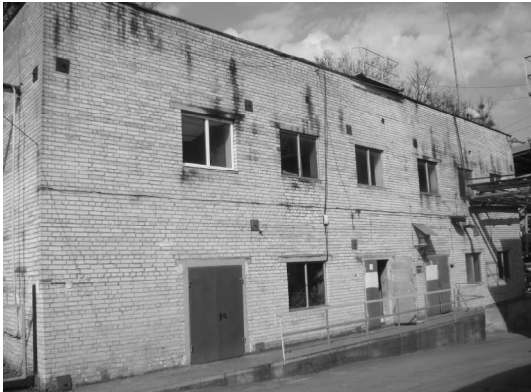
Photo 1. The main facade of the building ARS of axis "1" ... "3"
