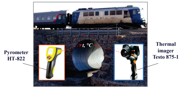
Fig. 1. The process of performing temperature measurements on the surface of a corrugated metal sheet of a pipe
