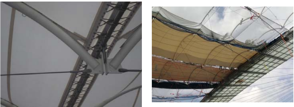
Fig. 14. Suspended arcs with stays tensioning the fabric and folding of the fabric – staff is visible
