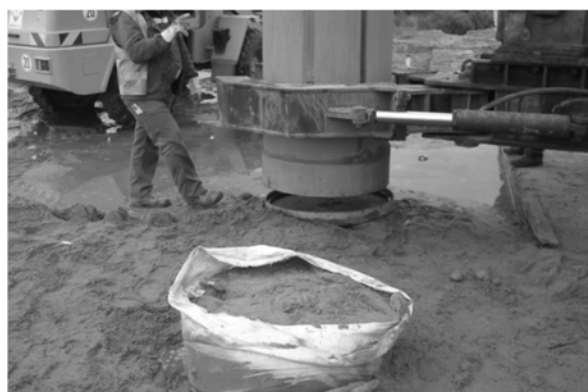
Figure 8 – Lost plate used at the base of the longest displacement pipes instead of standard flaps
