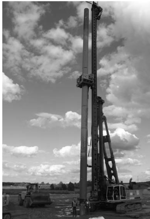
Figure 9 – Moveable ring vibrator used for the longest displacement pipes
