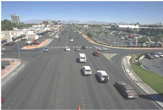
Figure 3 – A wide suburban street that was built without taking into account bicycle and pedestrian traffic (USA)
