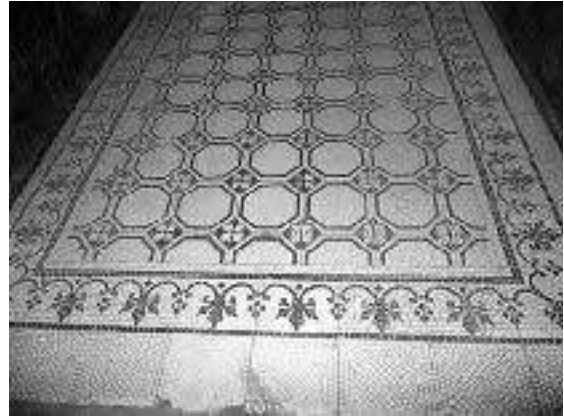
Fig. 6. Concrete tile with mosaic ornament in the house No. 14 on Kostya Levitsky street
