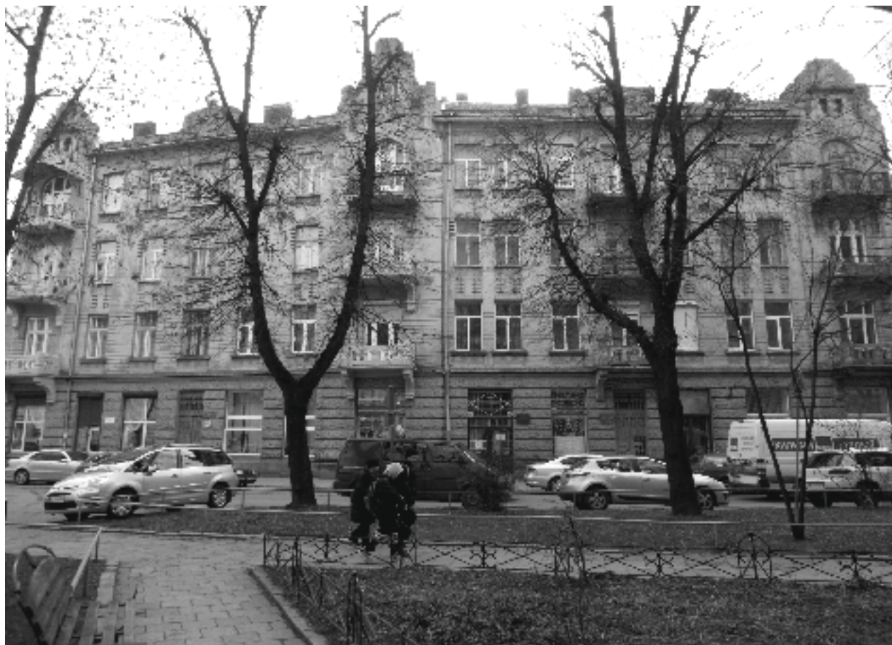
Fig. 1. The facade of residential buildings No. 14 and No. 16 on Kost Levitsky street
