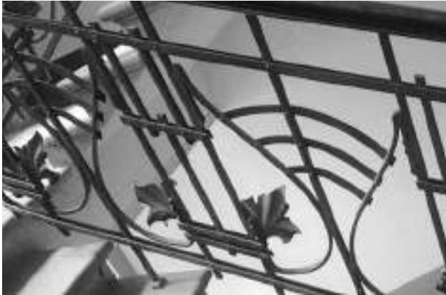
Fig. 5. Forged elements of the staircase of the house No. 14 on Kostya Levitsky street
