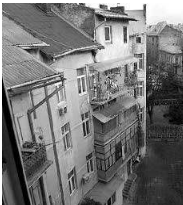
Fig. 9. View of the courtyard facade of house No. 16 from the balcony of the third floor of house No. 14 on Kost Levitsky street
