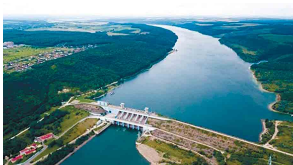
Fig. 2. General view of the Dnister HPP-1 and the reservoir [Online source: Official site of Dnister Water resources management].
