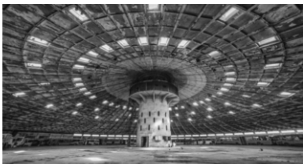
Fig. 27. Roof of bus fleet
