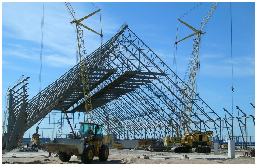
Fig. 3.1. Assembling process on job site (Photo has been provided by V. Shymanovsky Ukrainian Research and Design Institute of Steel Construction)
