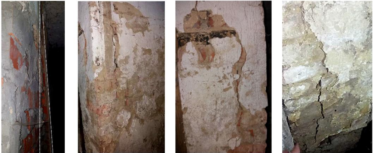
Fig. 3. Visible loss of resistance, as well as vertical and horizontal cracks in the middle bearing wall on axis B in axes 6–8
