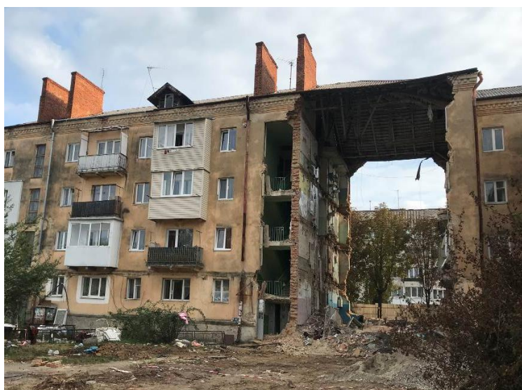
Fig. 2. The collapse of part of the building
