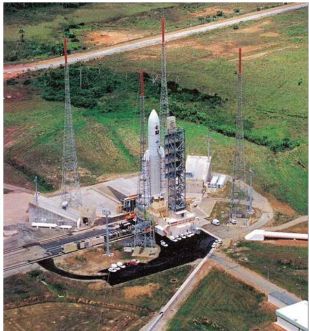
Figure 2 – Ground launch complex (appearance) [https://www.flickr.com/groups/ares/pool]
