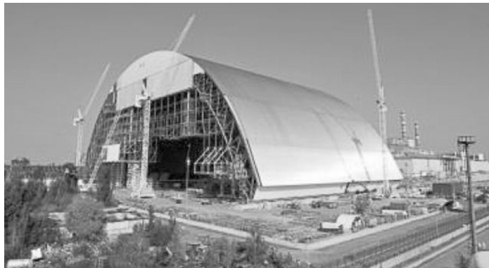
Fig. 4. View of the Chernobyl safe confinement (“shelter”) during its construction
